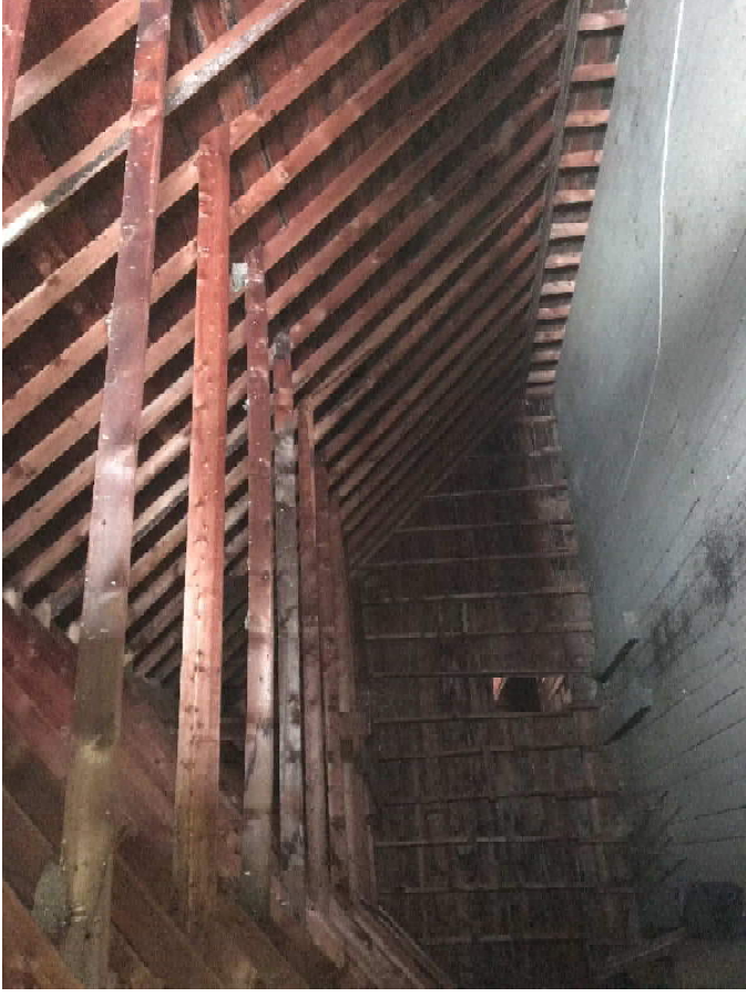
PHOTO 6: SCHOOLHOUSE ROOF FRAMING
