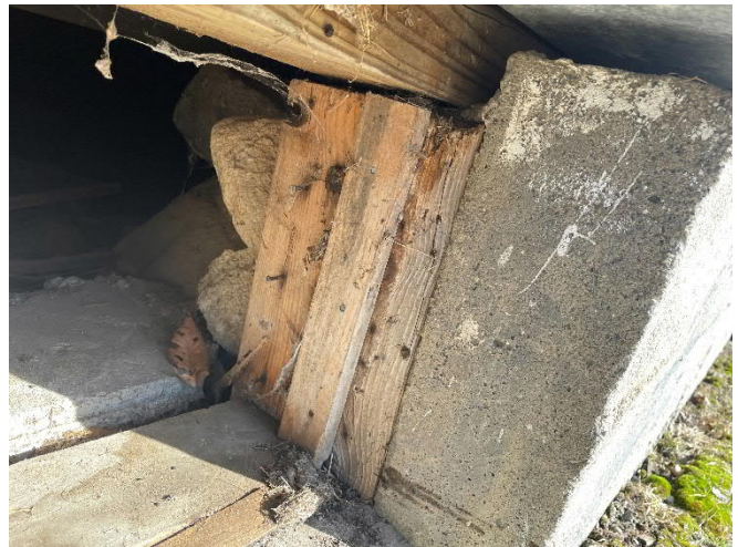
Figure 4 – Concrete over existing stone foundation
