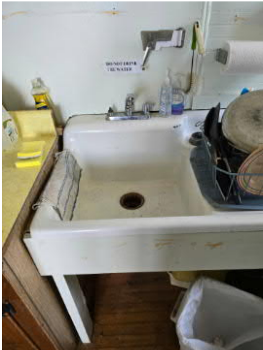
Figure 22 – Existing Kitchen Sink
