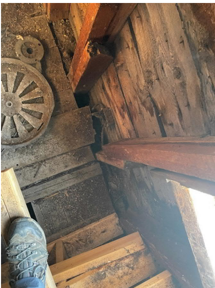
Figure 9 – Balloon framing visible from within the attic
