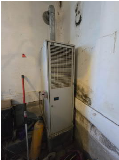
Figure 14 – Existing Wall Furnace
