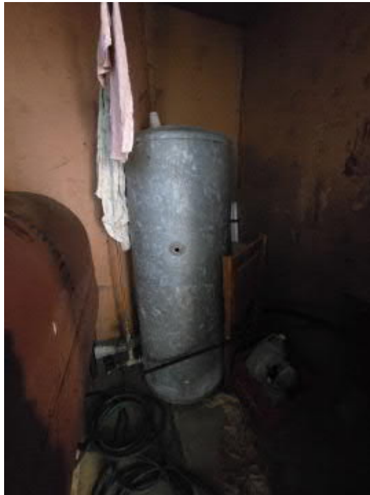
Figure 23 - Existing Water Tank
