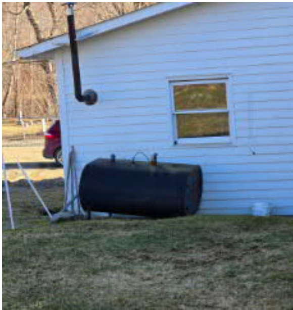
Figure 2 – Exterior Oil Storage Tank
